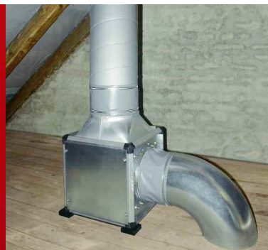
Installation in the attic with anti vibration mounts (accessories).
